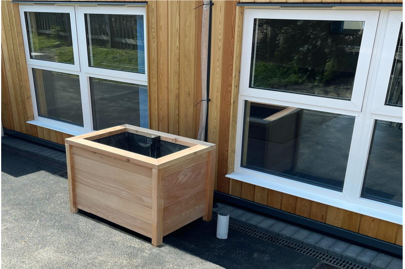
SuDS Planter in situ ready for connection
